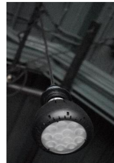
Figure 1 ZOBO lamps used as downlight pendants
